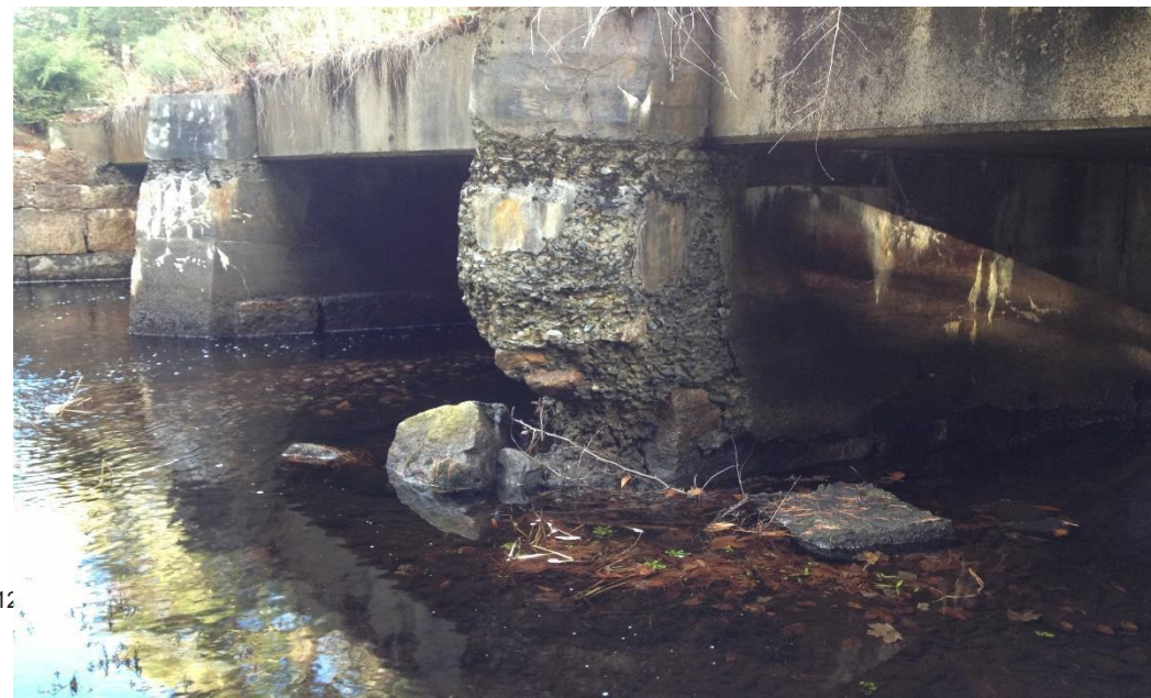
Examples of NHN Bridges Requiring Abutment, Pedestal and Repointing Repairs
