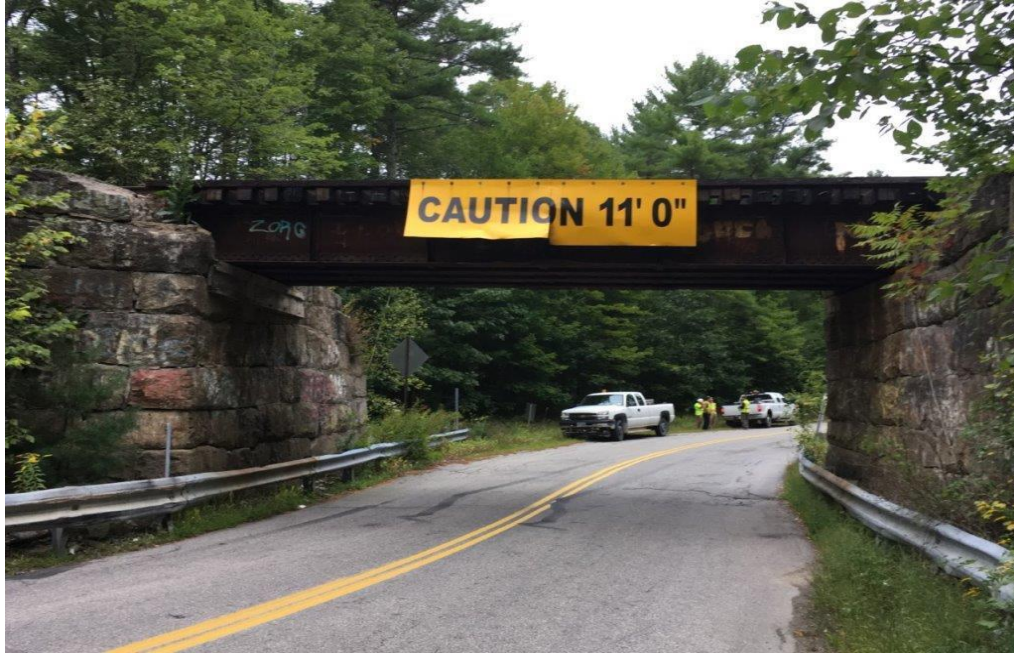
Examples of NHN Bridges Requiring Abutment, Pedestal and Repointing Repairs
